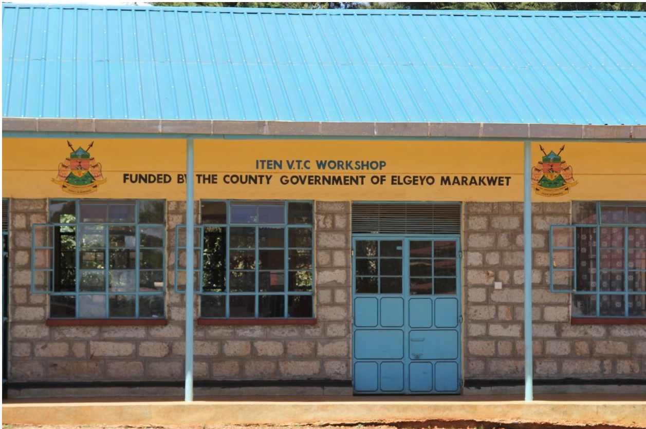
Figure 9. Upgrading of Iten VTC
