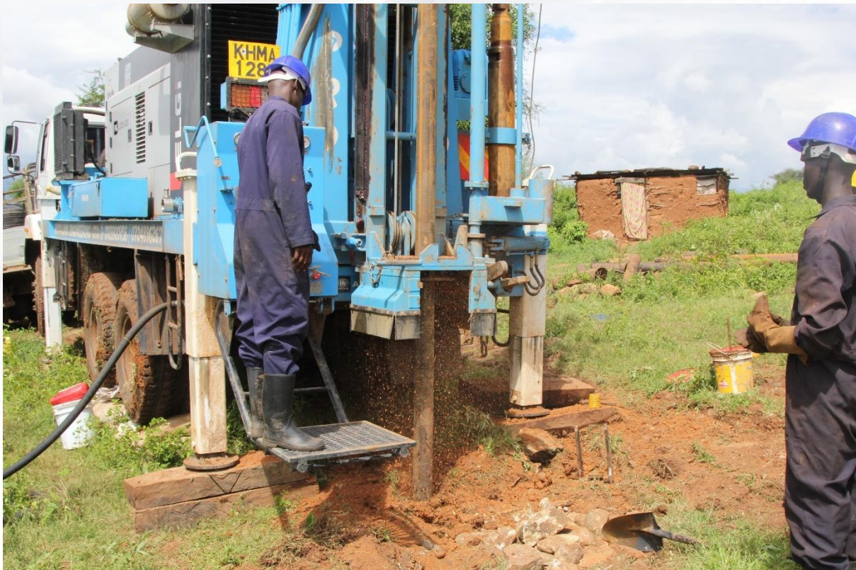
Figure 24. Drilling of Boreholes
